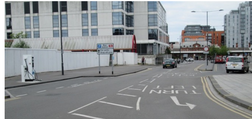
Rapid charger on Brunel Way opposite Slough Station Taxi Rank
